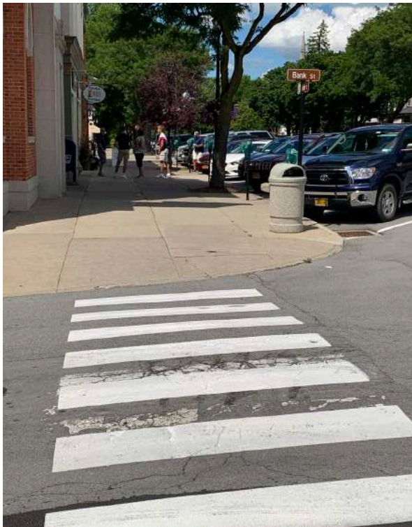
▲ Existing crosswalk in Geneseo. Curb ramp does not meet ADA standards but contains high visibility crosswalks.
