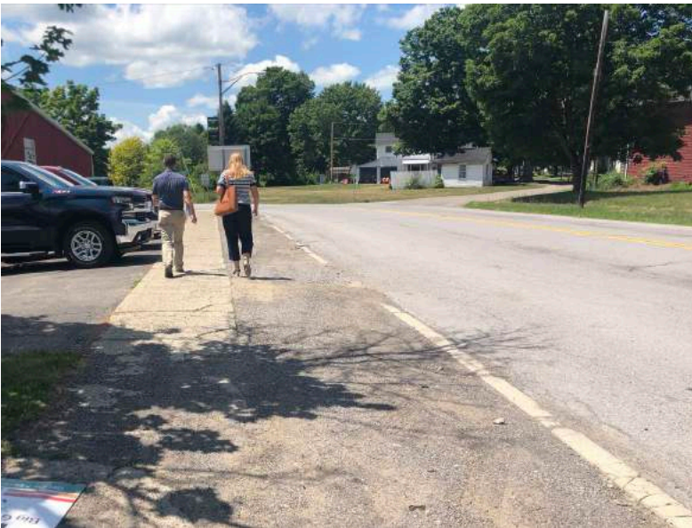
▲ In Nunda, gaps existing in the sidewalk connecting the Village to Kiwanis Park. There is also a lack of separation between the pedestrian and vehicular environment. (Image Credit: Google).
