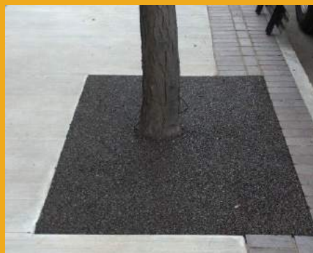
Flexi-Pave - A pervious treatment typically used in tree pits. This material is a good substitute for tree grates in narrow sidewalks where additional walking surface is desired.
