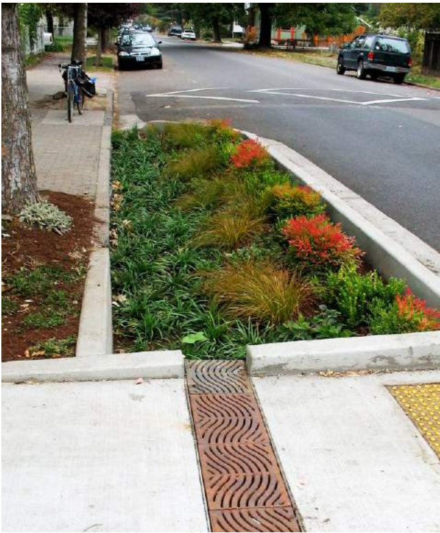
▲ Curb extension with green infrastructure in Portland, OR (photo credit: Justin Martin).
