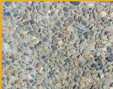
Exposed Aggregate Concrete - Used in the main path of travel and as an accent treatment.
