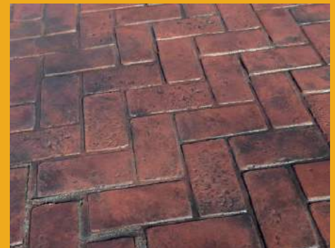
Stamped Concrete - Used as an accent pavement out of the main path of travel. Comes in a variety of colors and patterns.
