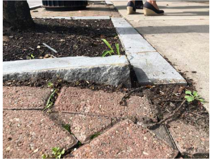
▲ Repair sidewalk and tree pit areas
