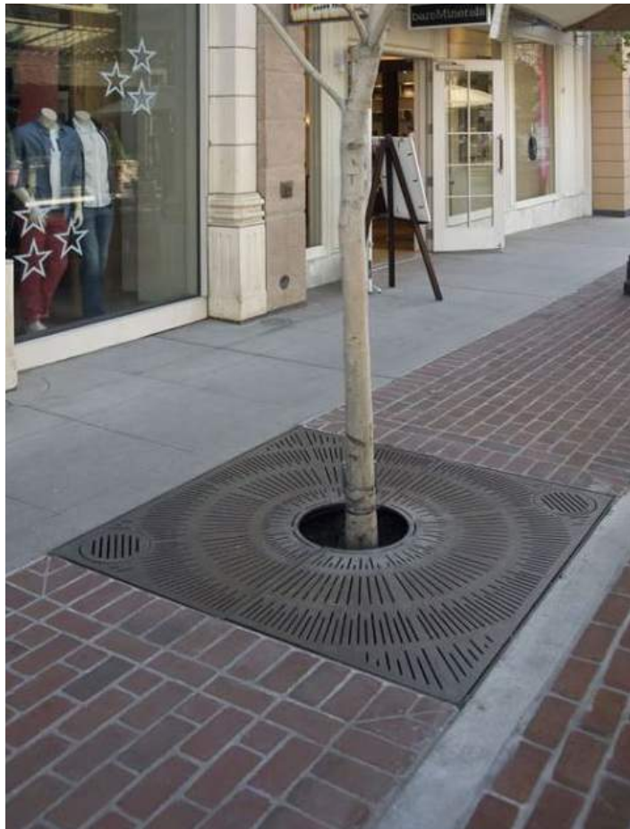
▲ Tree grates should have minimal openings to prevent the accumulation of litter and to provide an ADA accessible surface. Openings in tree grates should be no greater than 1/2" wide for ADA compliance (Image Credit: IronSmith).
