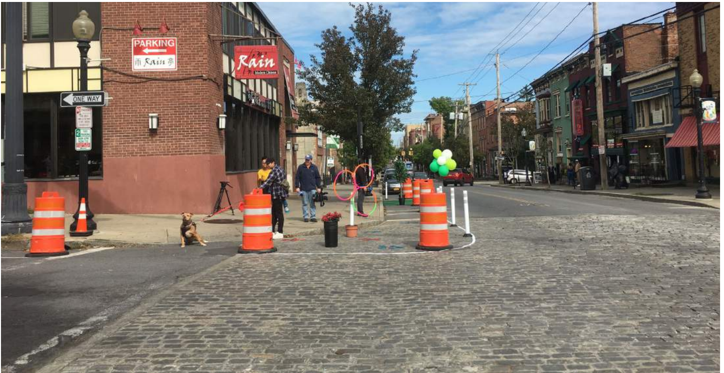
▲ Tactical urbanism demonstrations can be used to help educate the public on the benefits of curb extensions and test an idea before spending resources to design and construct. This image is from a demonstration project in Albany, NY; feedback from this exercise indicated that a 6 foot wide curb extension did not interfere with traffic flow and provided valuable pedestrian space.
