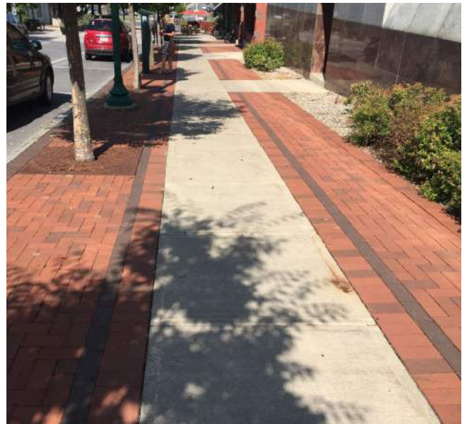
▲ A combination of materials can help add character to a Village sidewalk, while also defining use zones. The standard concrete in the center is the main path of travel. The brick areas to the side are amenity zones containing trees, light poles and site furnishings. The area to the left also provides an unloading area for parked cars.
