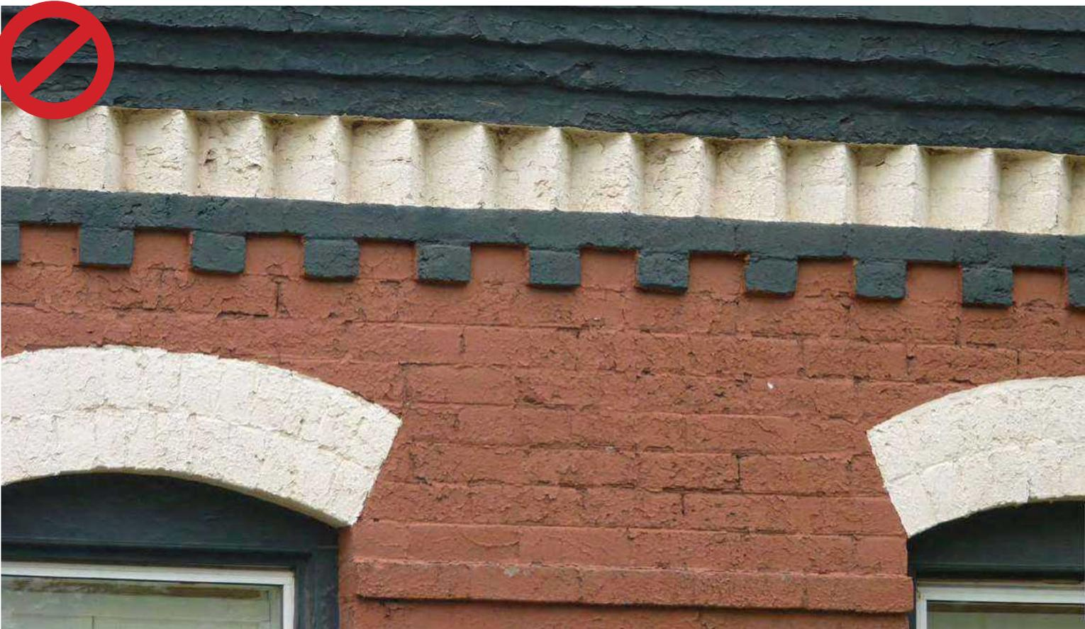
Repair aged masonry surfaces before repainting to avoid flaking paint with a reduced lifespan.
