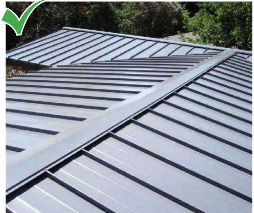
Use standing seam metal roofing for a durable replacement.
