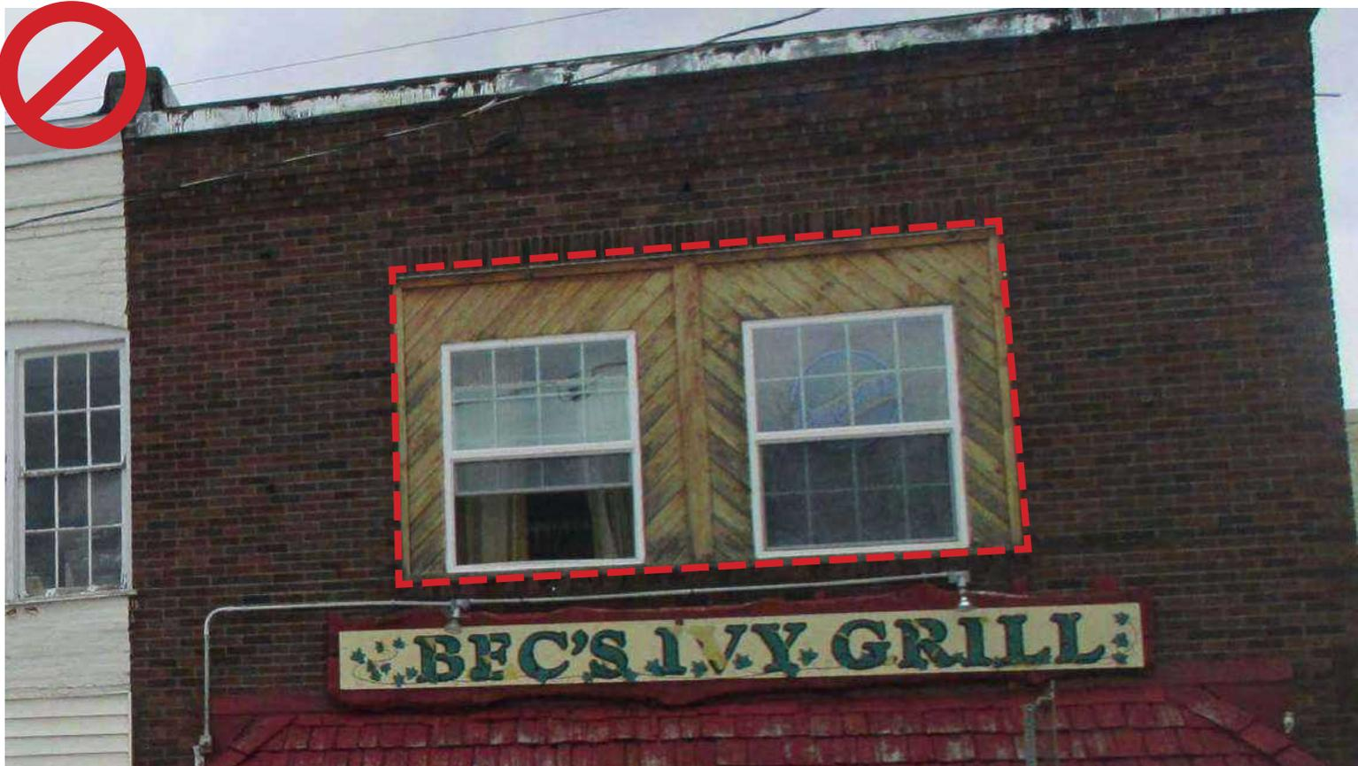
Do not fill in large upper floor window openings with smaller, undersized vinyl windows.
