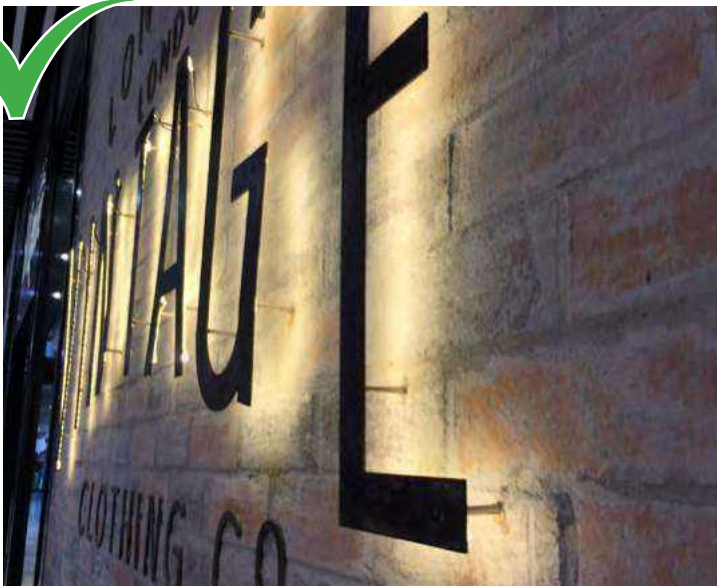
Signage must utilize exterior lighting - such as this halo-lit sign mounted to an existing masonry wall.
