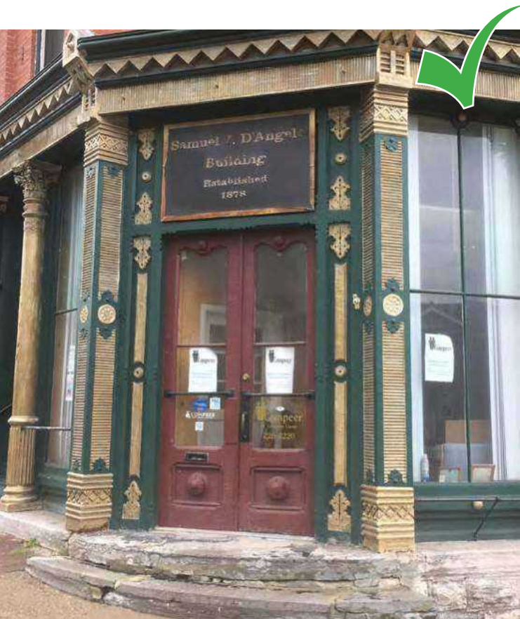
Restore and maintain historic entry doors.
