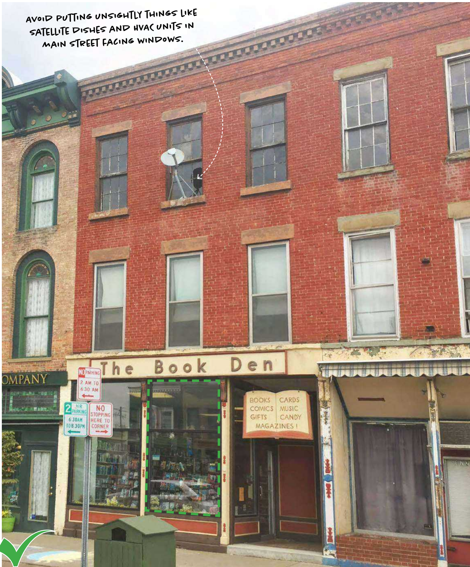
New window replacements should be sized to match existing opening sizes to maintain historic visual access
