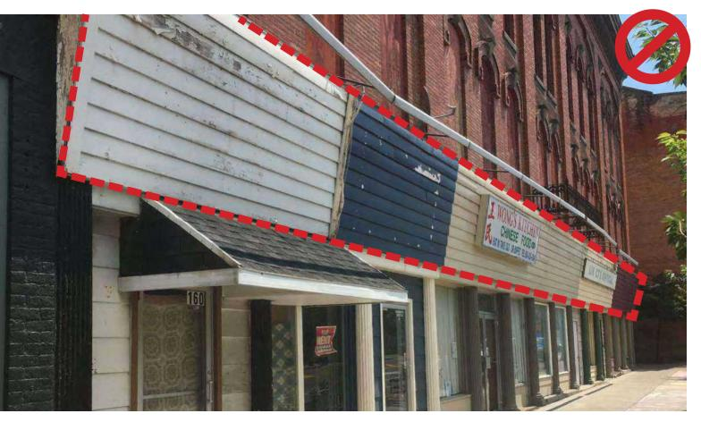
Do not cover original materials such as masonry or wood cladding with inappropriate materials such as stone veneers or vinyl siding. Do not cover up original storefront openings and details.
