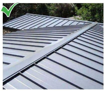
Use standing seam metal roofing for a durable replacement.
