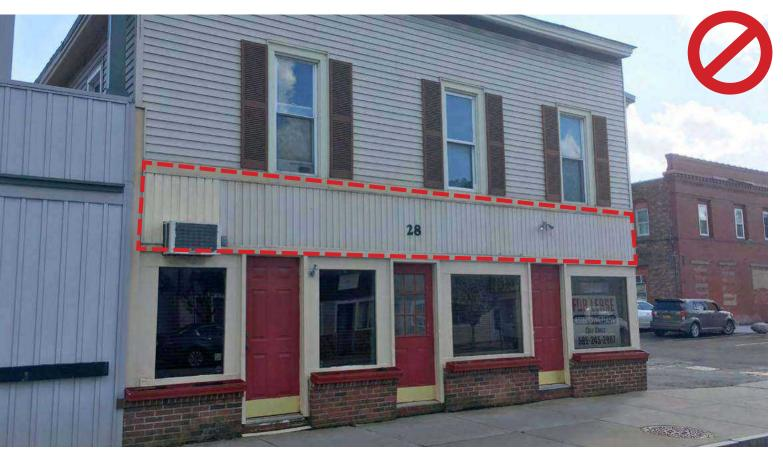
Do not use vinyl siding to replace transom window details. Do not use vinyl replacement windows with inappropriate sash and frame profiles. Do not use residential HVAC window units.
