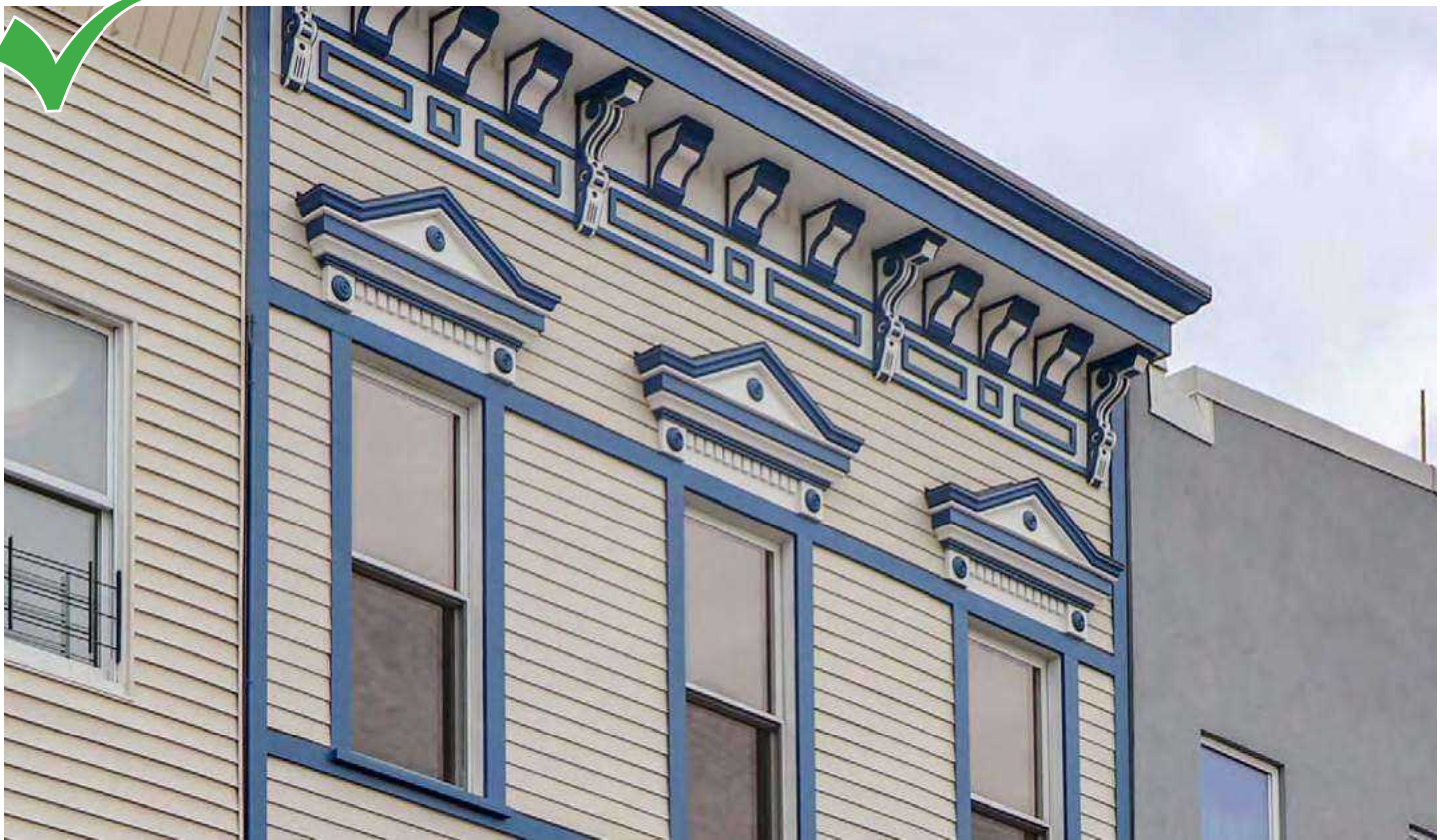
Use materials that can be repaired and maintained - such as fiber cement panels and siding. Fiber cement can be used to replace wood that has reached the end of its lifespan.
