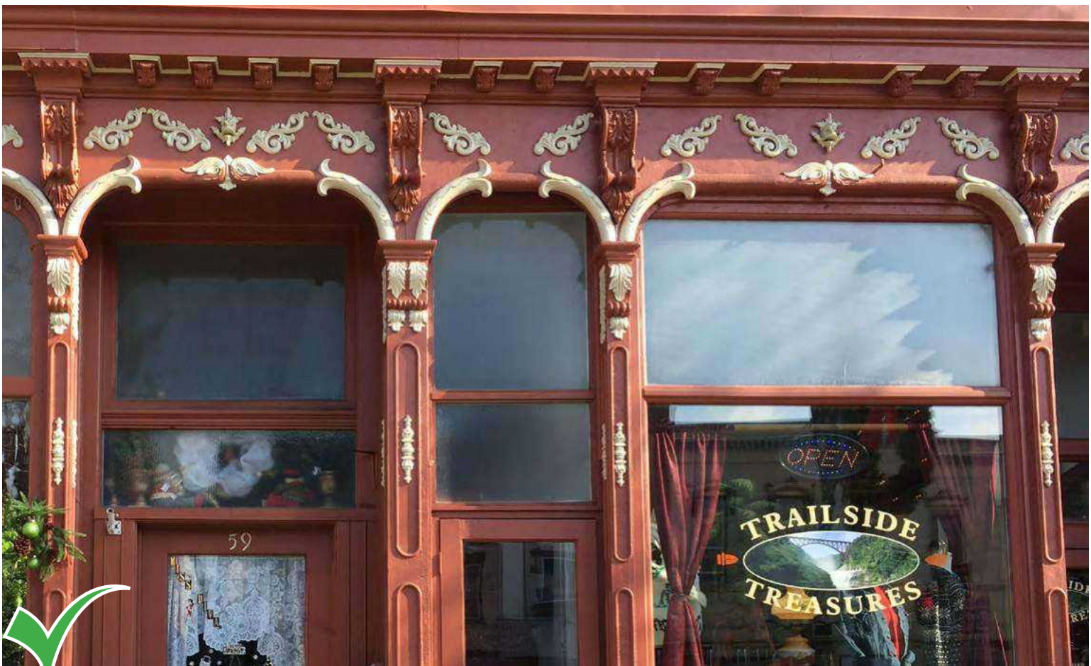
Uncover and restore original steel columns and cornice detailing.
