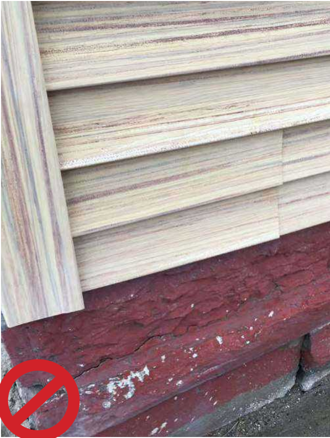
Do not use residential vinyl siding or paint a fake wood grain on it to mimic wood siding.
