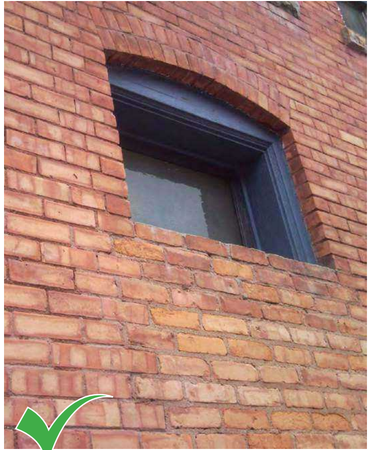
Repair and restore original materials when possible.
