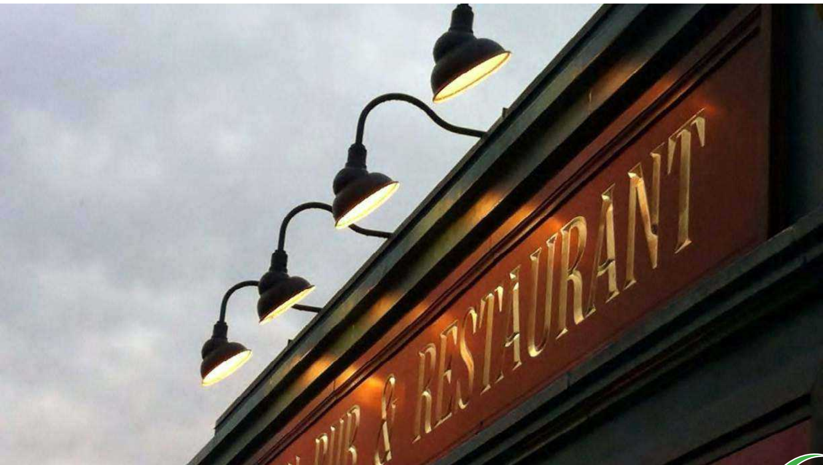
Ensure lighting fixtures provide an even spread of light onto the signboard.
