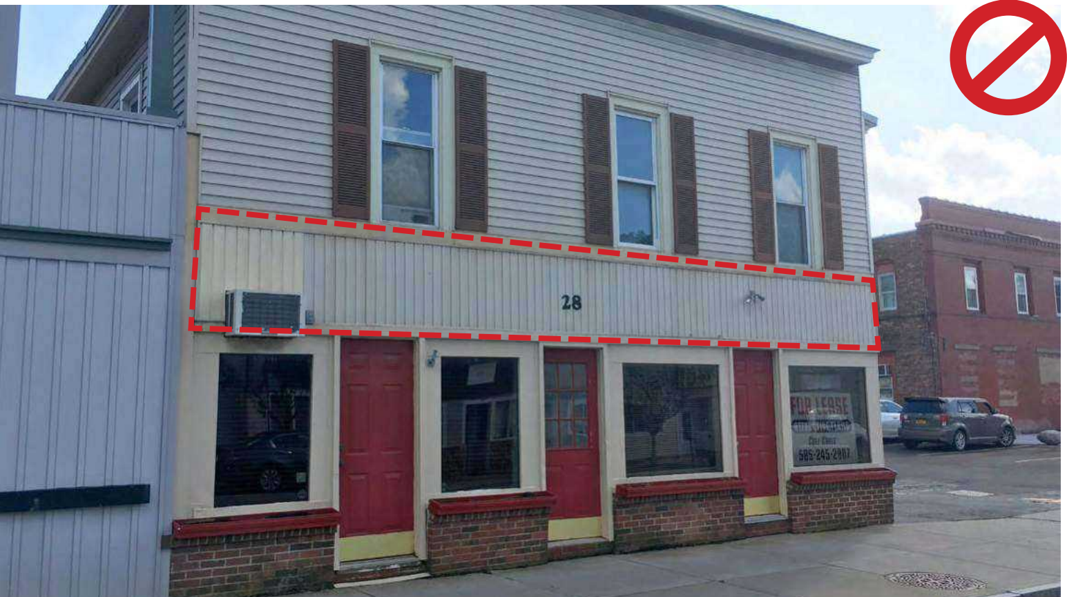
Do not use vinyl siding to replace transom window details. Do not use vinyl replacement windows with inappropriate sash and frame profiles. Do not use residential HVAC window units.
