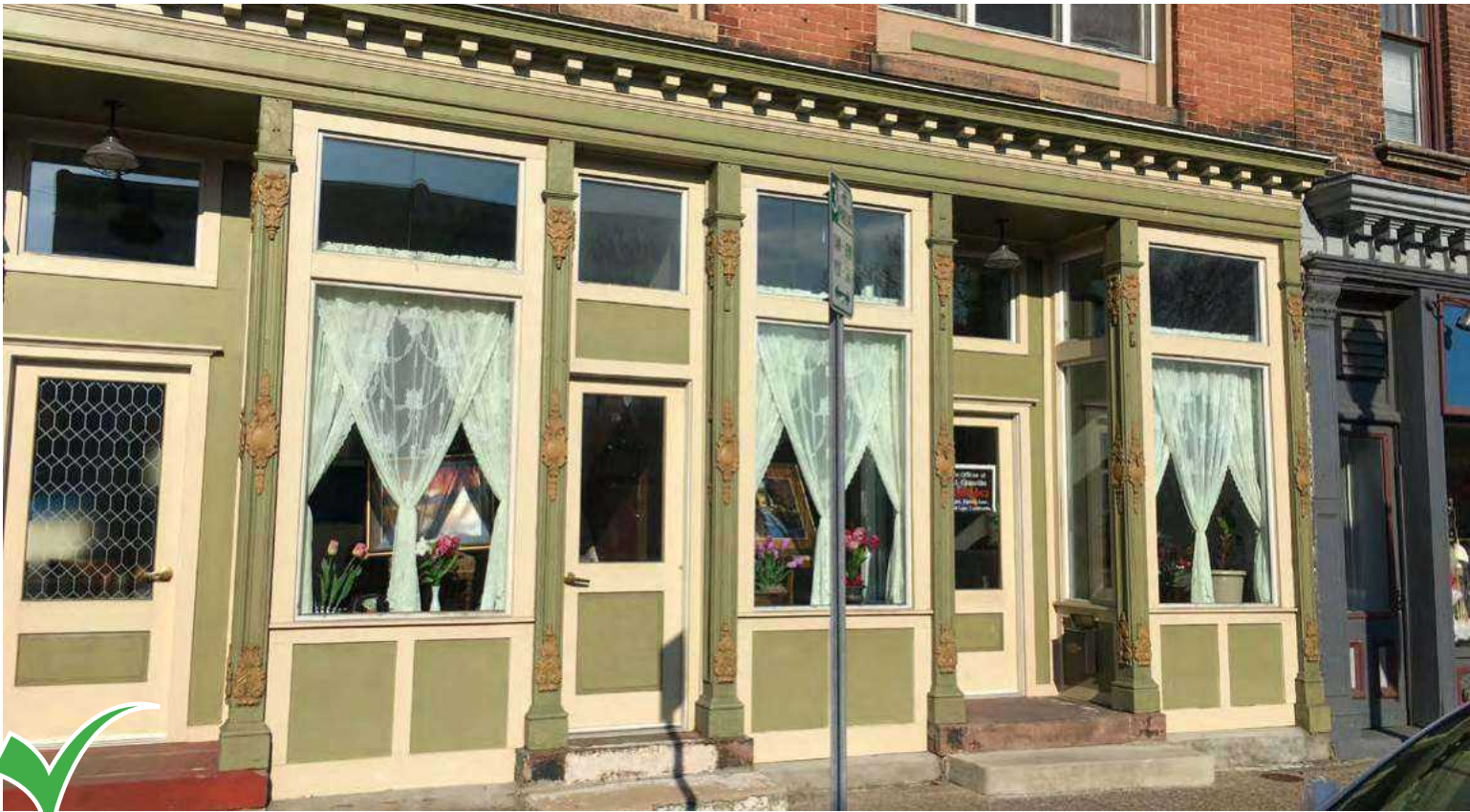
Use appropriately sized window sill and sash profiles when specifying replacement windows.
