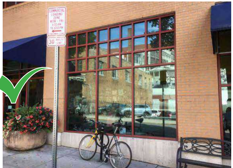
Use a variety of window patterns and sizes on replacement windows to bring down the scale of large openings.
