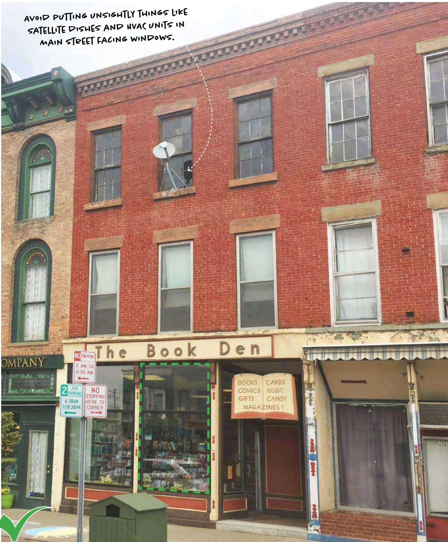
New window replacements should be sized to match existing opening sizes to maintain historic visual access
