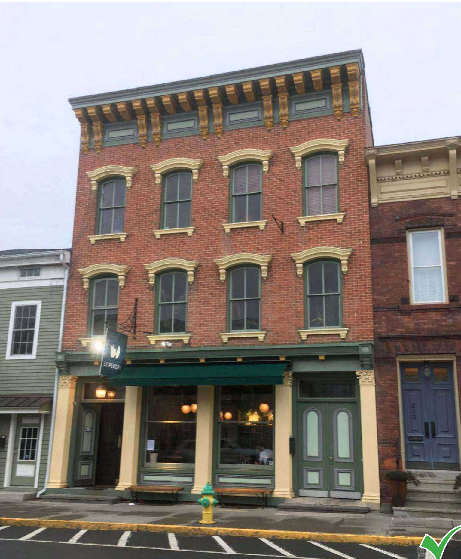
Highlight historic masonry details such as lintels, window sills, and columns with paint to both protect and highlight them.
