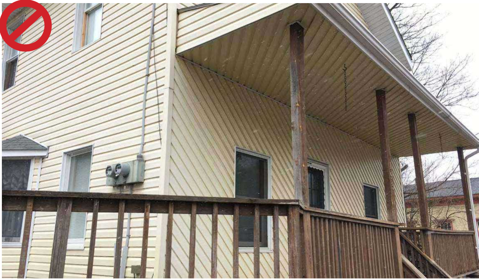
Do not cover up existing wood siding with prohibited materials such as vinyl or metal siding.
