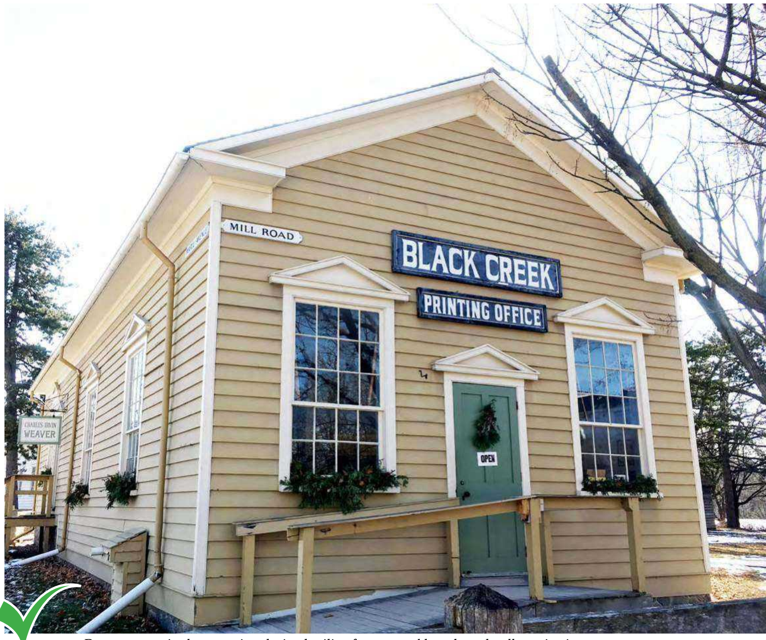
Do use appropriately proportioned trim detailing for eaves, gable ends, and wall terminations.
